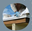
use of re-enforcing Poly Fabric on all roof joints, penetrations and surface overlaps to ensure a seamless roofing surface..
